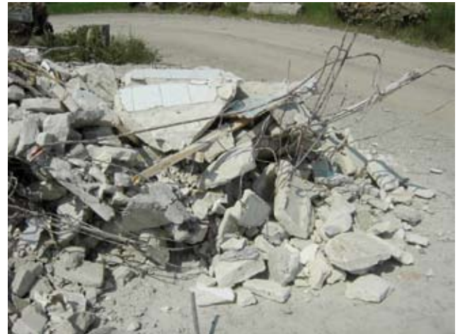
11 Gipsbaustoff aus der Badzelle Building material from the bath cubicles
